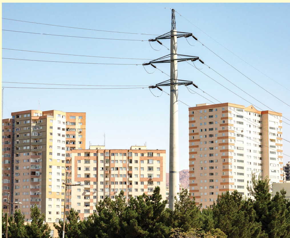
132 kV Line on Tavanir Street, Tabriz Serving as the eastern ring of metropolitan Tabriz, constructed using Pars Sakhtar's self-supporting single-pole concrete towers.
